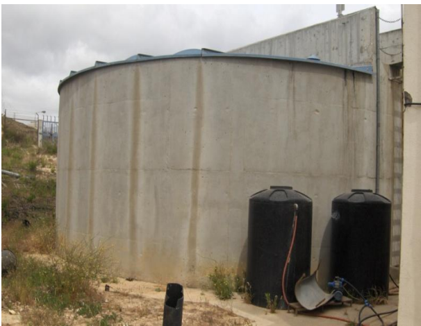
Photo 1.2: Sludge Thickener tank at Al Bireh WWTP
