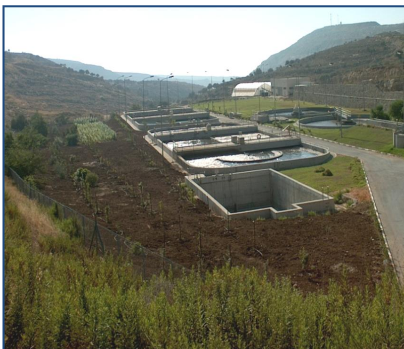
Photo 1.1: Al-Bireh Wastewater treatment plant
