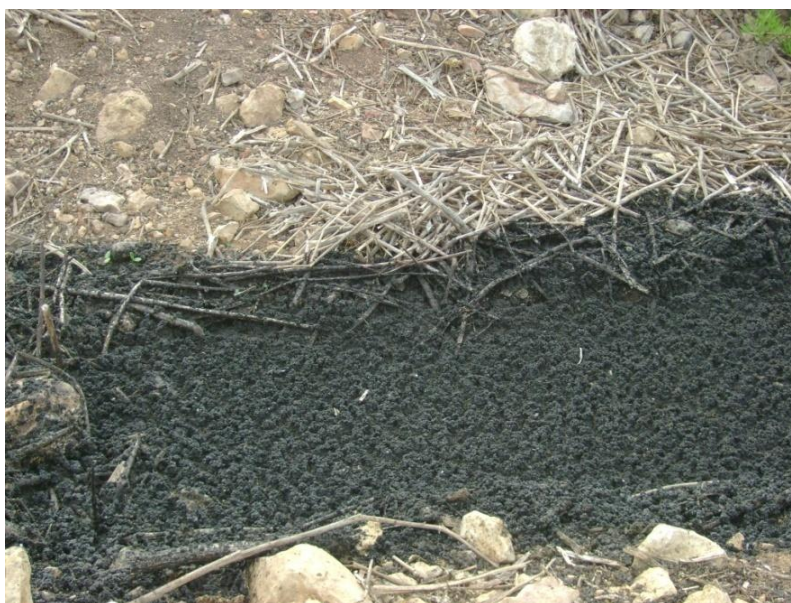
Photo 3.13: Sludge drying process
